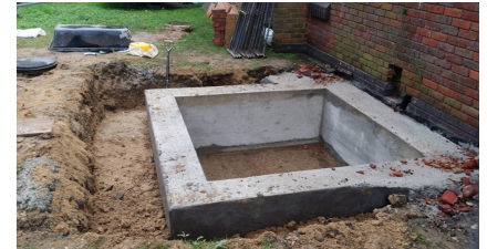
Concrete pit under construction
