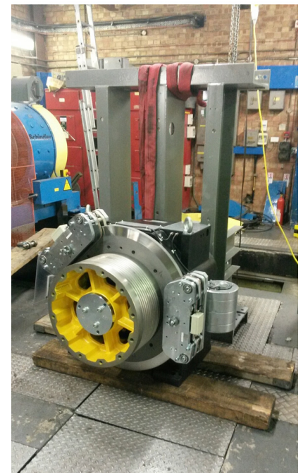
Replacement gearless drive unit being installed
